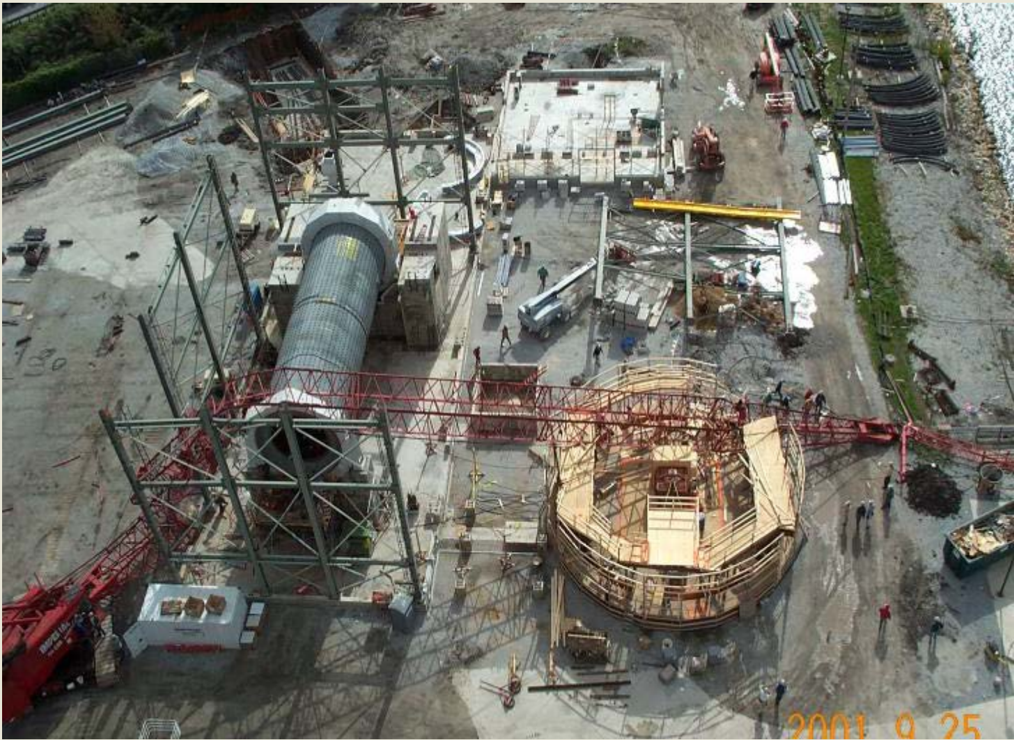
The crane boom after it buckled due to overload because of excessive lift radius.
