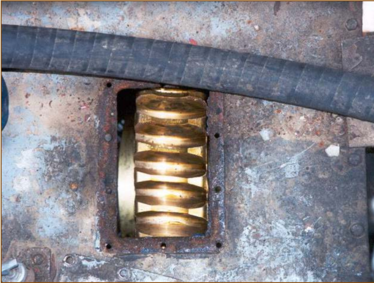
Boom hoist gearbox inspection.
