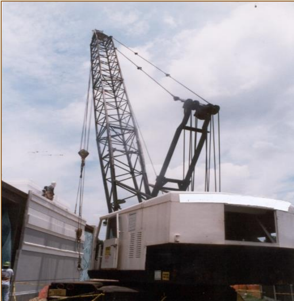
A friction crane that had its boom drop during a routine lift.
