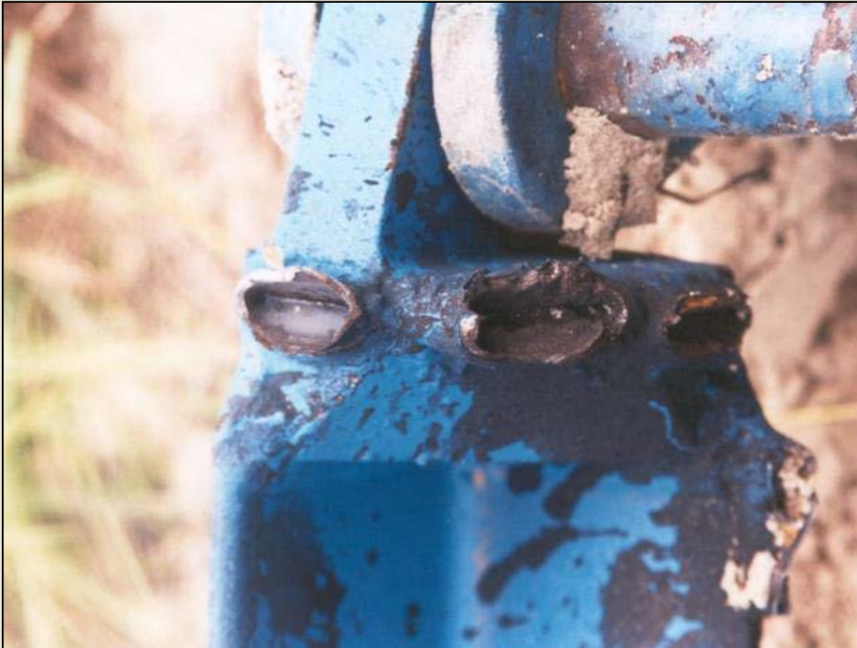
Lattice boom fracture surfaces that were caused by a boom overload.
