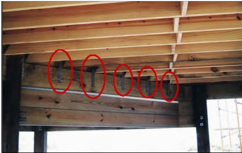
Typical floor framing connections. (FEMA News Photo)
