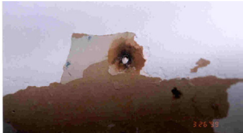
FIGURE 7 Niceville, Florida. Heat damaged drywall covering the wood blocking where the cheese melter hanging bracket lag bolt penetrated the wall.
