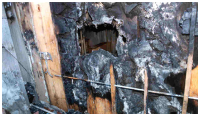
FIGURE 5 A close up view of the origin area depicted in Fig. 1. The burned hole through the wall corresponds to the heat pattern on the back of the cheese melter.
