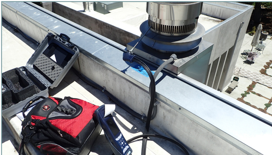
Field testing of flue gas
